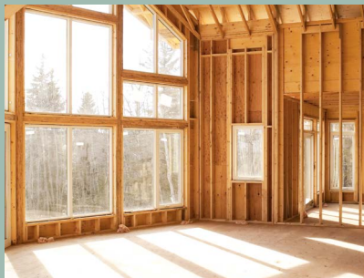
Manufacturing windows and doors
