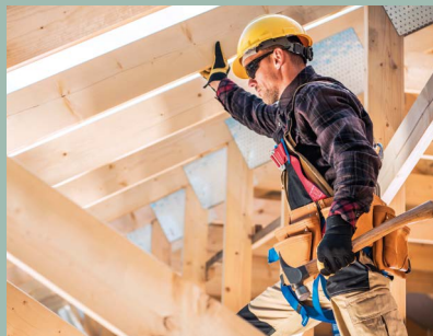
Roofing houses, windows and doors
