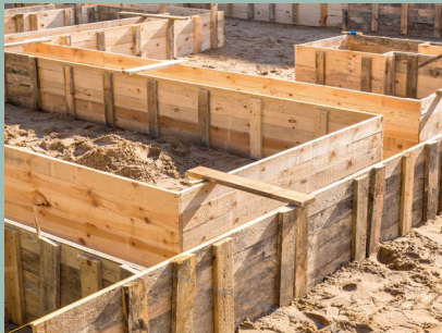
Scaffolding and formworks
