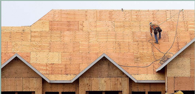
Exterior and interior decoration works
