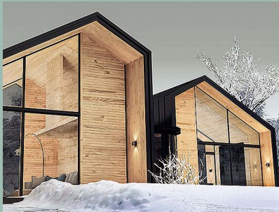
Exterior decoration of buildings
