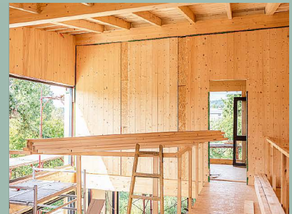
Exterior and interior finishing
